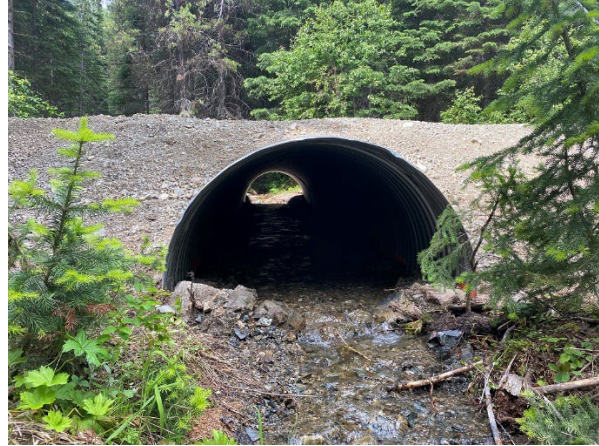
Figure 2: An example of a 2-foot culvert replaced with a half-buried 6-foot diameter culvert. The high velocity of water in undersized culverts restricted fish passage and increased the chance of a catastrophic failure. The new culvert allows for higher stream flows and improved fish passage.
