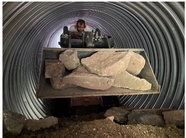
Figure 3: The installation of a culvert includes removing the old culvert, setting the pipe at grade, and placing streambed material in culvert to allow for easier fish passage. Finally, the entrance and outlet are armored and revegetated with transplants and native seed.
