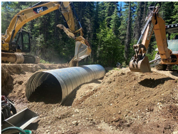
Figure 3: The installation of a culvert includes removing the old culvert, setting the pipe at grade, and placing streambed material in culvert to allow for easier fish passage. Finally, the entrance and outlet are armored and revegetated with transplants and native seed.
