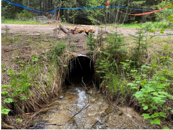
Figure 2: An example of a 2-foot culvert replaced with a half-buried 6-foot diameter culvert. The high velocity of water in undersized culverts restricted fish passage and increased the chance of a catastrophic failure. The new culvert allows for higher stream flows and improved fish passage.
